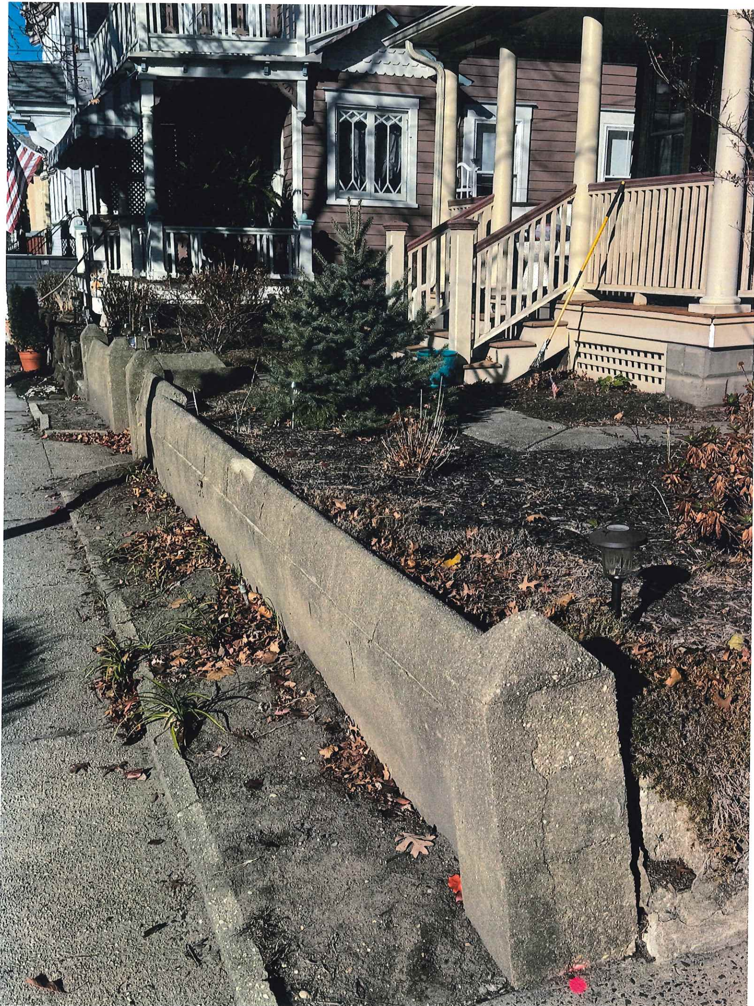
95 COOKMAN Existing Retaining Wall
