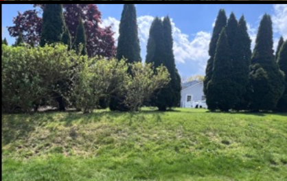
E: Subject Site Building
