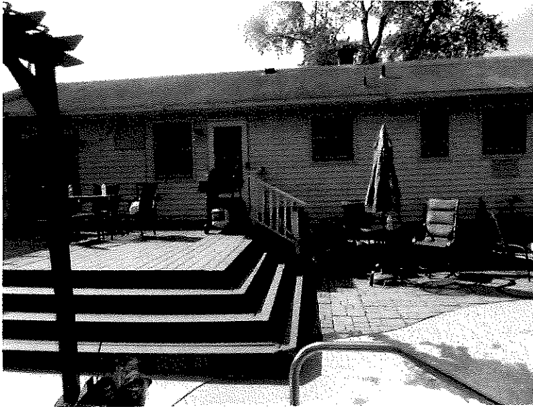
Photo 5 Steps wrapping around back left corner of deck.
