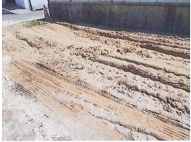
Removed west UST
