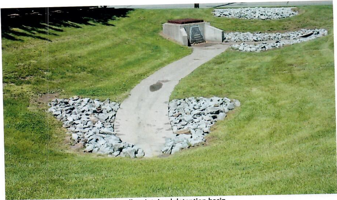
A well maintained detention basin
