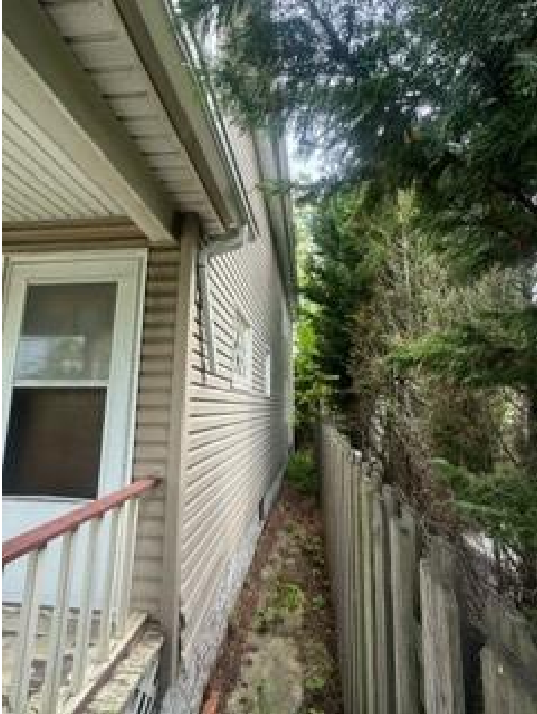
Side (West Facing)
