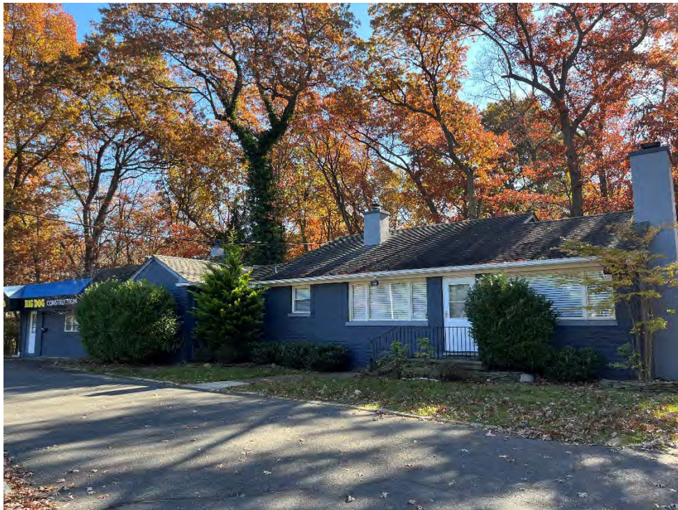
Figure 2: Existing structures presently located on site
