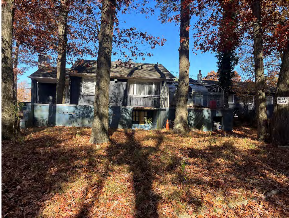
Figure 3: Rear of structures located on site
