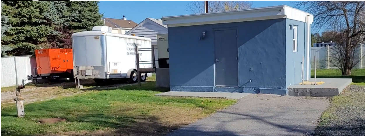
View of the Existing Sanitary Sewer Pump Station Building and Department Equipment.
