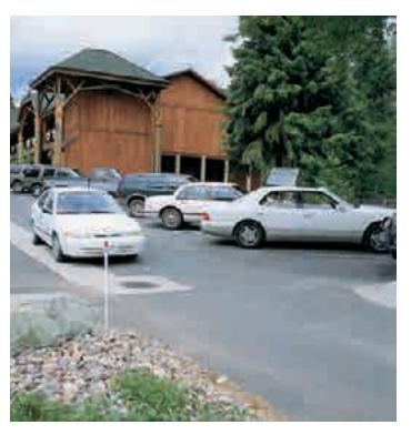
Above: Two views of a completed RS<sup>3</sup> install under a parking lot in Big Fork, MT. Parking lot and off-street bays for approximately 48 cars, drains into a 26,250-gallon Rainstore<sup>3</sup> stormwater detention structure. Diagonal parking is graded toward the center concrete strip, which drains toward the catch basin.
