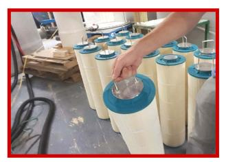
Once Cleaned Install Back Into the Vault. This Completes Maintenance. Ensure Access Lids are Properly Replaced.
