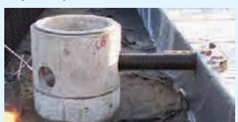
Inlet and pipe interface with Rainstore<sup>3</sup>
