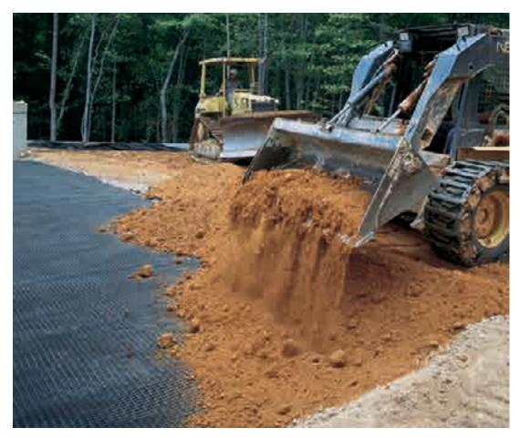
Left: Heavy equipment begins to put the cover material over an installed Rainstore<sup>3</sup> chamber. Take extreme care when driving and/or compacting over the chamber and do not drive over exposed Rainstore<sup>3</sup> units — wait until ALL the units are installed, the side backfill is complete, fabric and geogrid layers are completed, and an adequate amount of cover material is placed.
