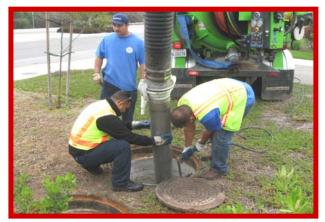
Remove Access Hatches Set Up Vacuum Truck to Clean The Pretreatment Chamber.
