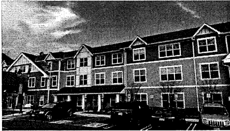
Illustration E.8.a. — Reference photograph showing modern double and triple window fenestration as found in a non-historic area residential structure. Note the use of a standing-seam roof in this contemporary example.
