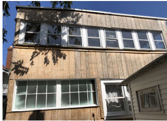
VIEW #1 (REAR WALL) T1-11 PLYWOOD CLADDING
