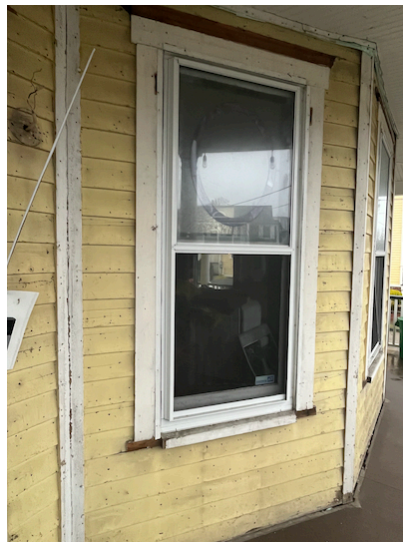
front/north elevation (note cut sills)
