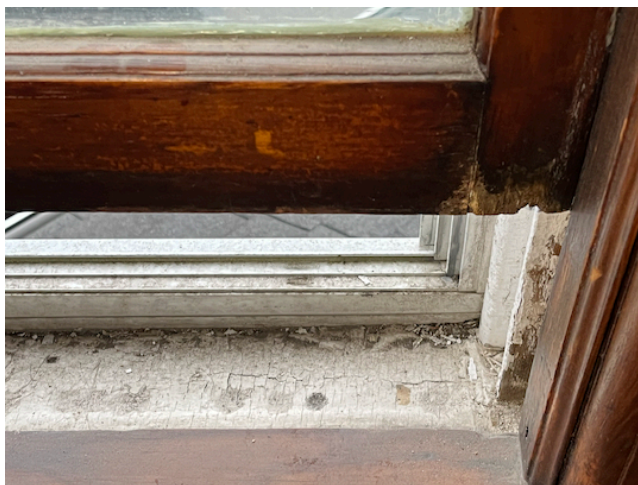
window 2-6 with detail of lower left sash (perhaps the most damaged)
