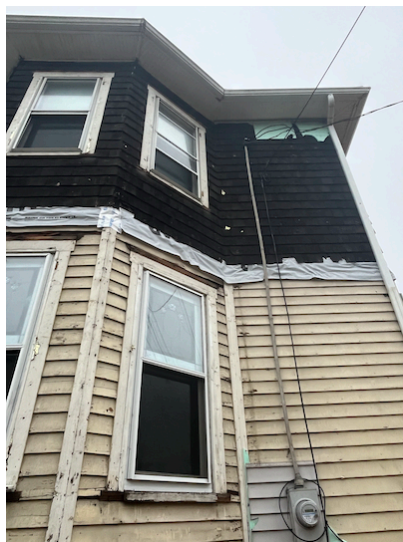
west elevation towards south; note damaged window surrounds
