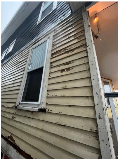
northeast corner with damaged clap; note cut sills/missing crowns
