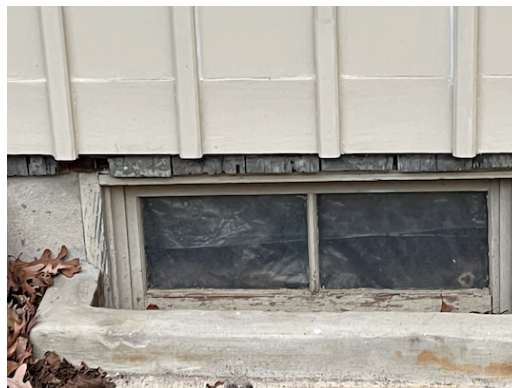
south elevation with newer board and batten on top of deteriorated board and batten
