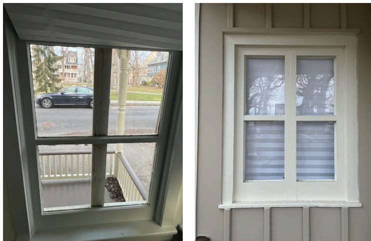
single window facing north appears to be a casement to the exterior and a 1/1 on the interior, both fixed in place.
