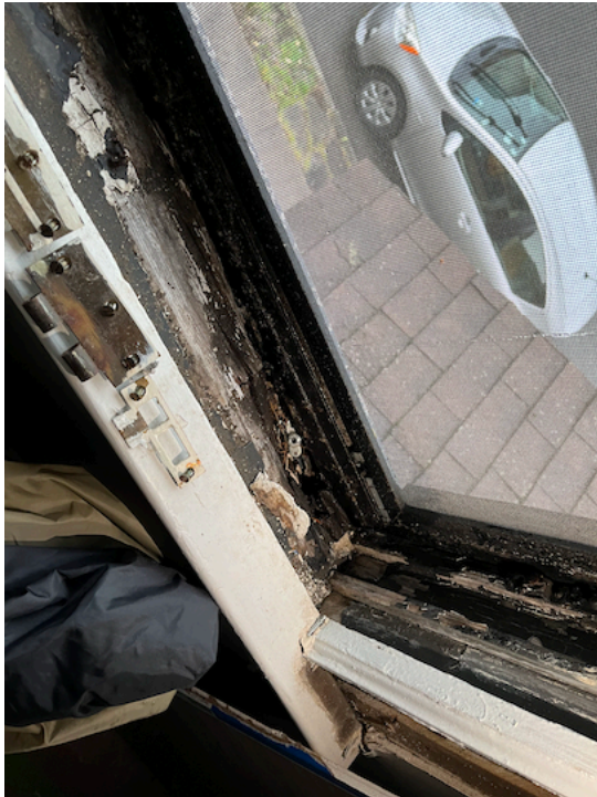
rot in sills of two second-floor windows
