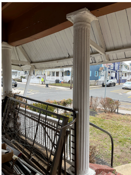
Column #2: poor (abacus split/rotted; column split at railing connection)
