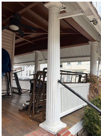
Column #2: poor (abacus split/rotted; column split at railing connection)
