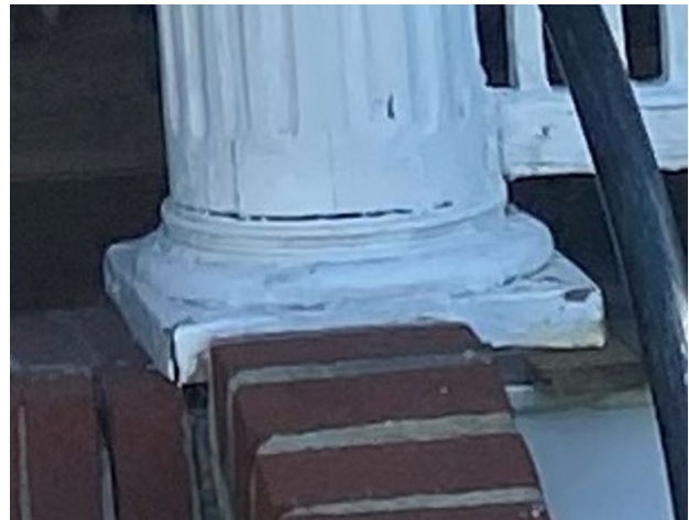
CLOSE UP OF DETERIORATED COLUMN BASE
