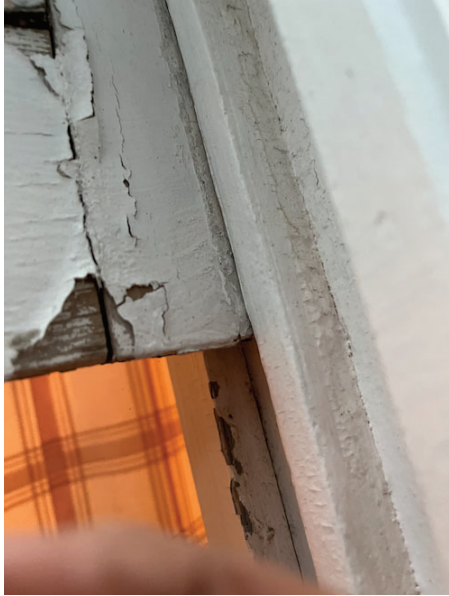
exterior of window on east side showing splitting sashes
