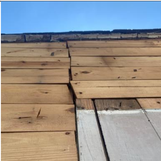
13: newer sheathing boards at recent additions
