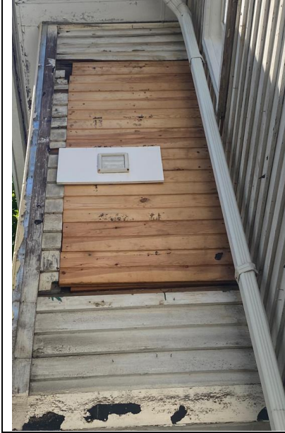
15: window opening infilled with newer sheathing boards
