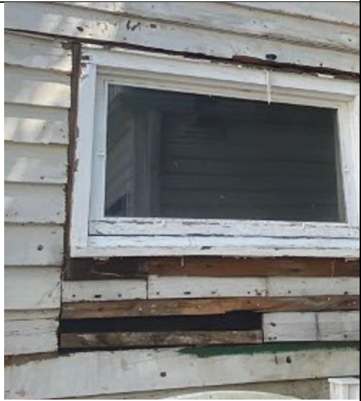
4: patching around window opening. clapboard cut to accommodate window installation.
