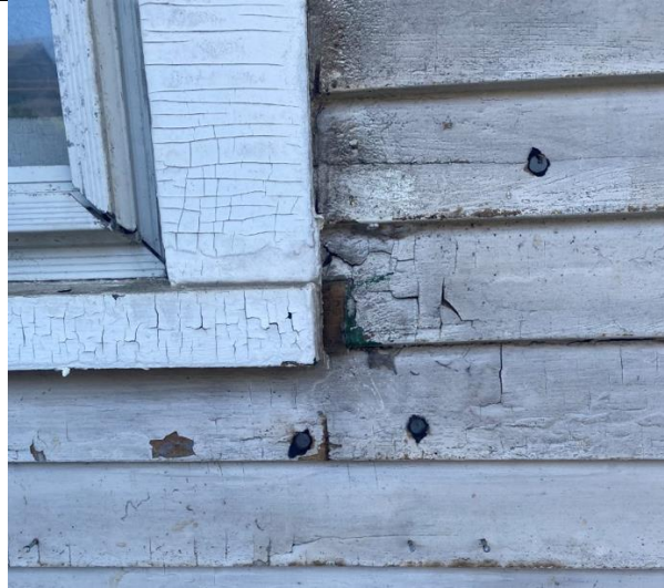
2: Sill extension cut to accommodate asbestos siding installation.
