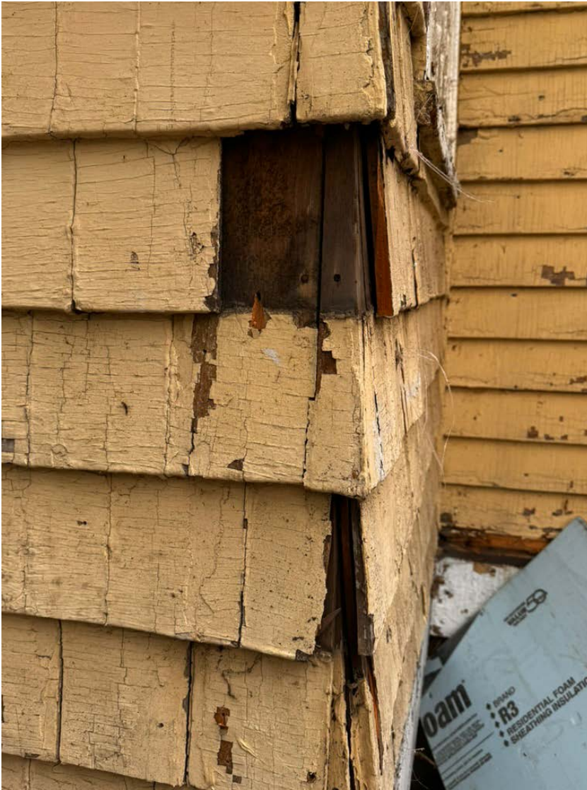
A detail of shingles at one of the woven corners.
