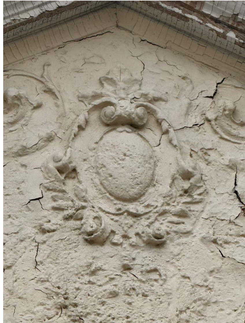
Original plaster bas-relief ornamentation in the pediment over the entry stairs is crumbling. The underlying supports appear to have been undermined by years of water penetration into the plaster and horsehair material.
