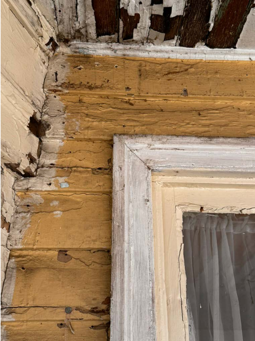
At the north elevation, under the porch roof (and area normally protected from weather and water) signs of severe damage near the roof indicate water penetration from above.
