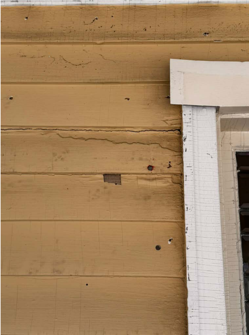
In a small area at the north elevation, beneath the porch roof where the clapboard is not obviously split, there are signs of pronounced cupping, suggesting underlying water penetration.
