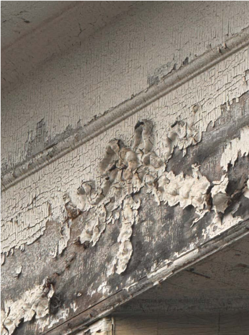
The bas-relief ribbons and swags of the ornamental frieze are almost complete deteriorated, with elements completely missing in areas where material has flaked off and been lost. The wood appears to have mold in areas.
