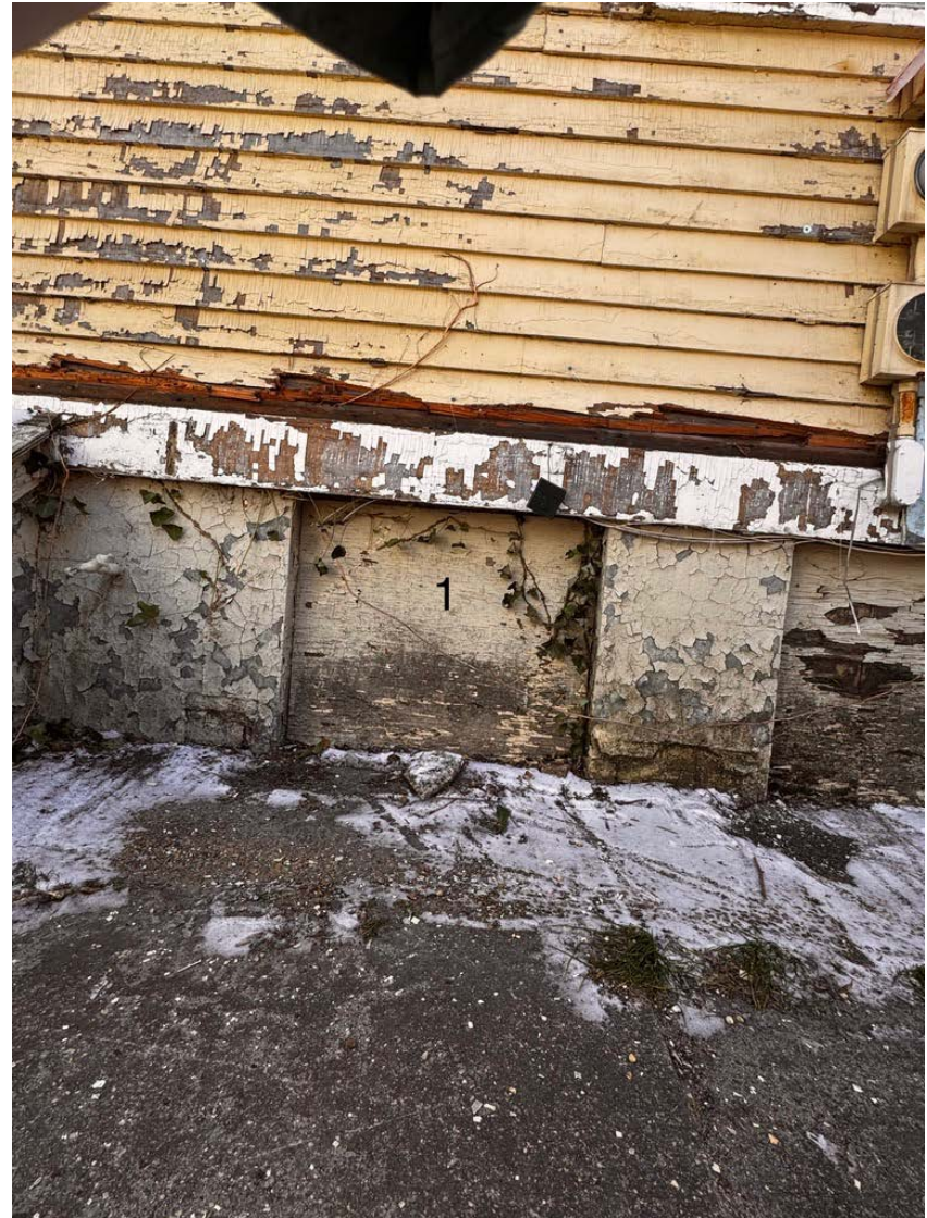
The west elevation is representative of the condition of clapboard throughout: split, cracked, cupped, and spongy with moisture (wet and fibrous as seen in the lowest course of boards, above).
