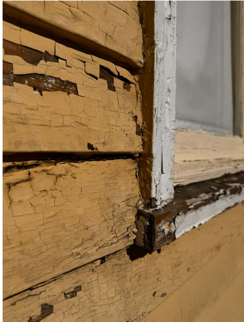
In areas clapboard has dried and shrunk so much the boards no longer overlap.
