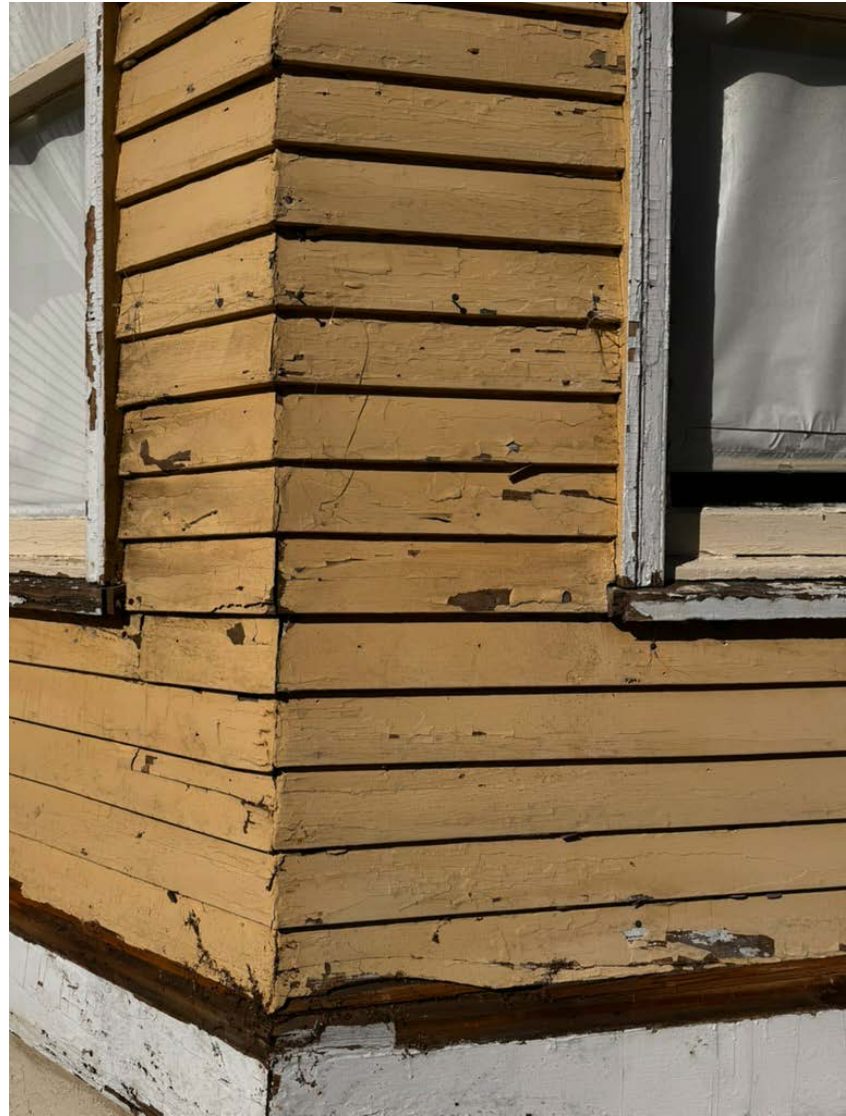
A detail of the woven corners. Such craftsmanship is found on both the east and west bays.
