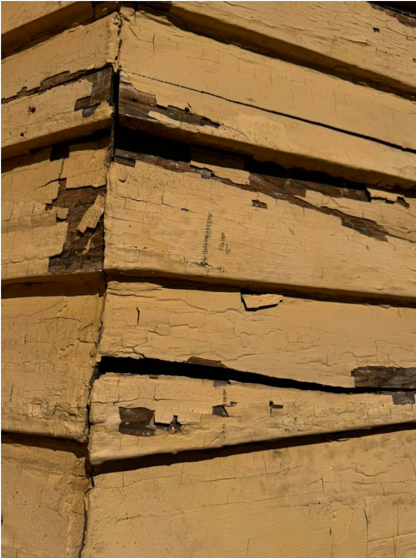
At the west elevation which gets the worst weather and blazing evening sun, the damage is even more pronounced with large gaps opening across the entire elevation
