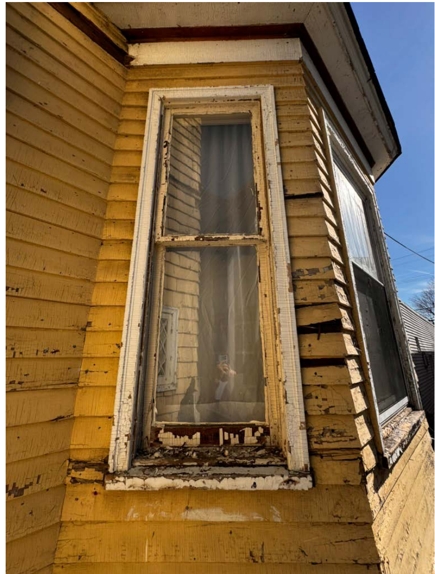
Window, trim, and cladding share a similar degree of decay.
