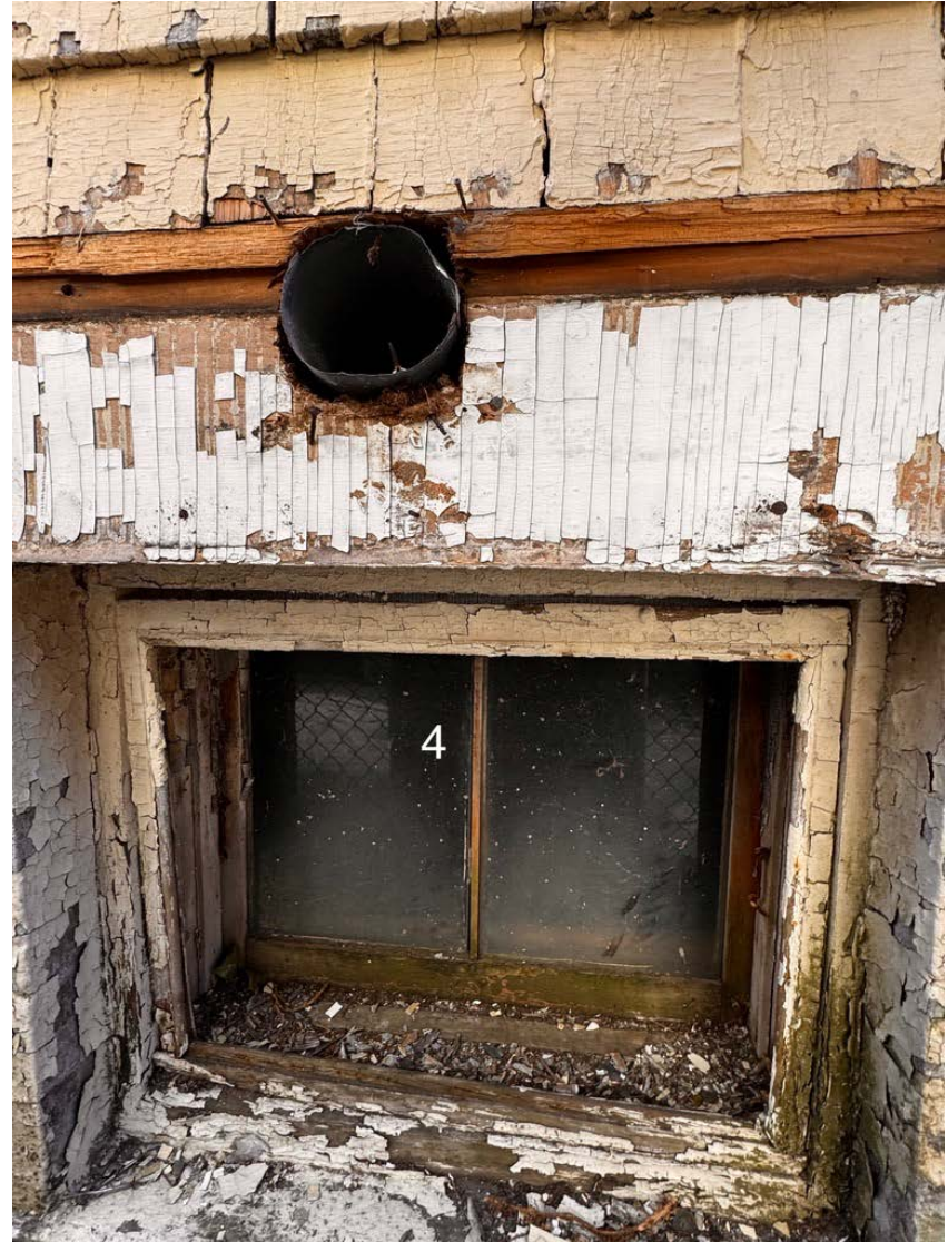
A detail of the condition of one of the basement windows.
