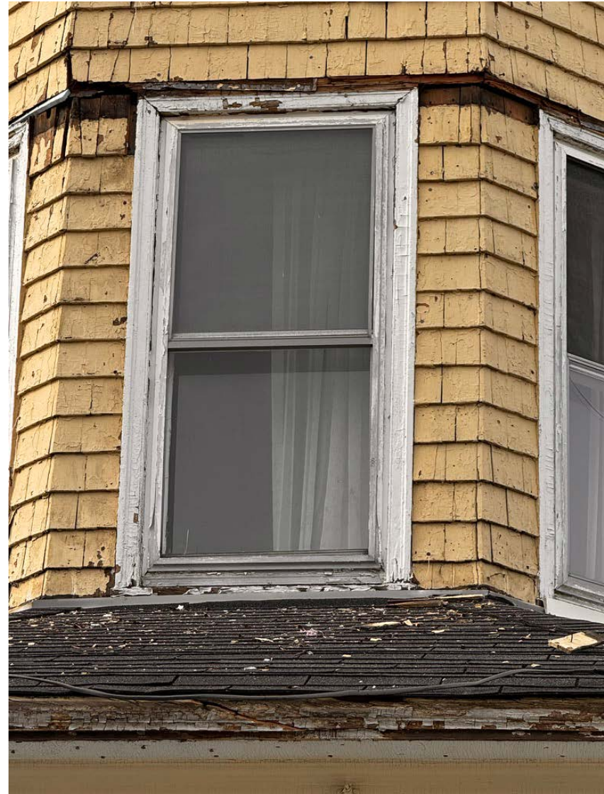
Closer inspection revealed multiple coats of paint disguising the countless split shingles and rotted wood.
