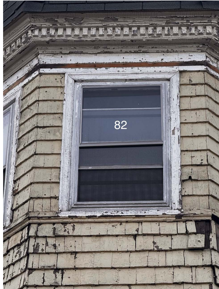
A view of the Level 3 tower showing deterioration in the crown and dentil molding beneath the dome of the turret.
