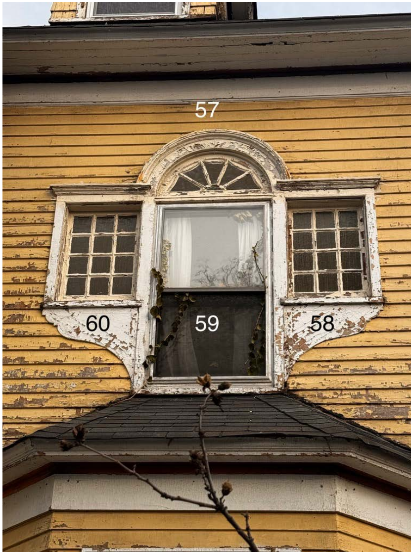
The trim around this ornamental window-set at the west elevation is rotting. Water is also penetrating behind this trim from the rotted sill pans.
