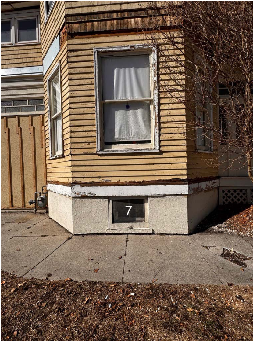
Level 1 of the east elevation bay. Note how clapboard is woven at edges around the bay bends.
