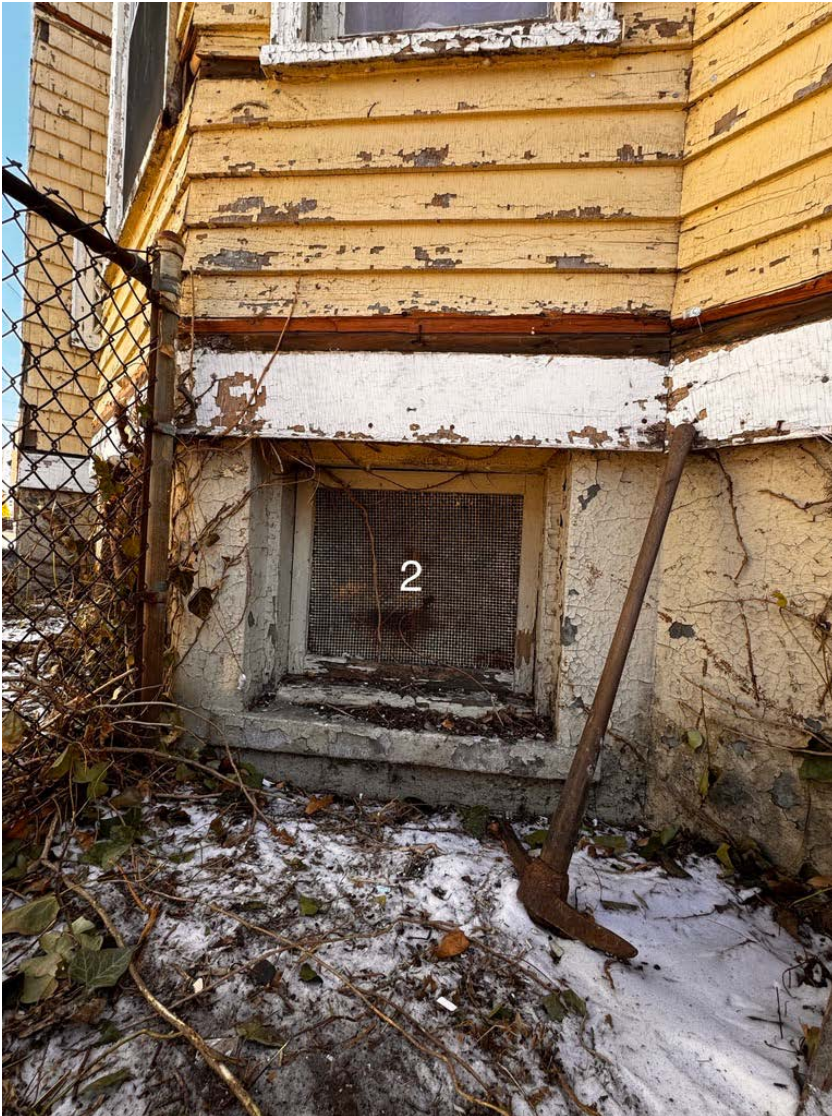
Lower cladding revealed to be wet after removal of vinyl cladding. Parged foundation is cracked in areas and basement windows rotted in the frames.
