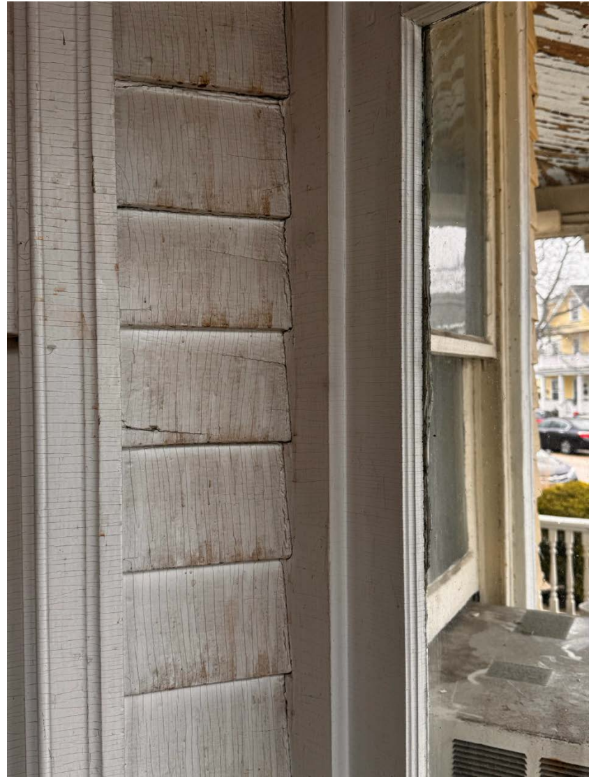
A short run of siding in the enclosed portion of the porch, though protected from weather, still show signs of deterioration caused by water penetration from turret windows above.
