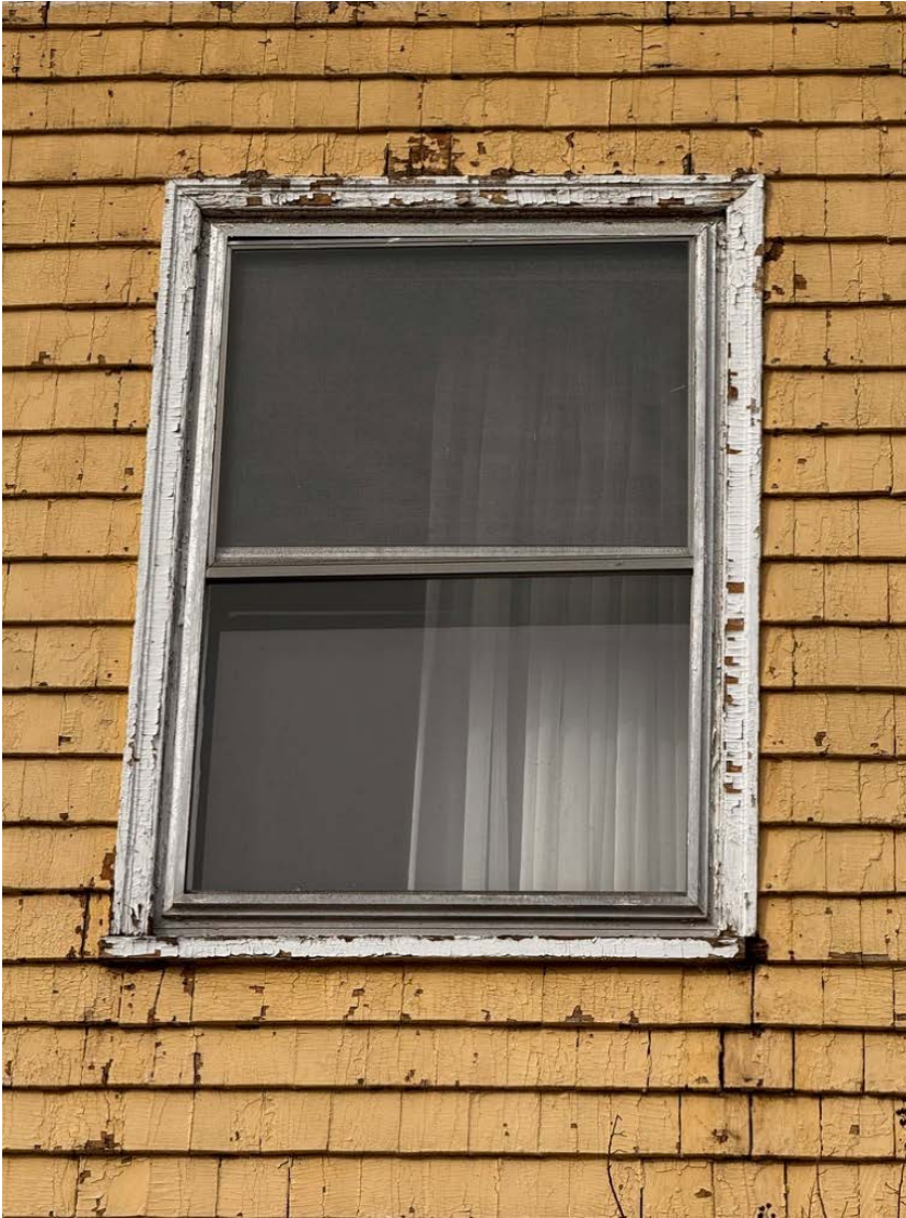
Severely cracked and rotted shingles are held together and in place by many layers of old paint. Non-conforming, non-original, mitered window trims of indeterminate age are broken, rotten, and have had all of their sill ears lopped off.
