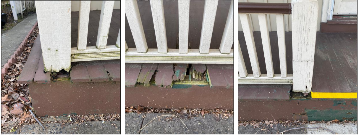
Evidence of rot and deterioration of the 1 st Floor Porch
