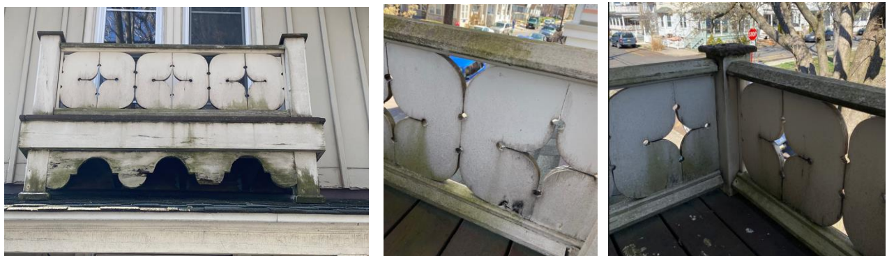
Evidence of rot and deterioration of the 2 nd Floor Balcony's wood components
