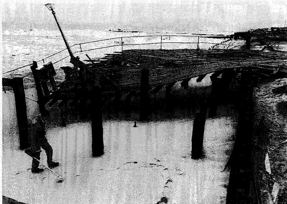
Section of boardwalk in Ocean Grove damaged following storm in December 1992
