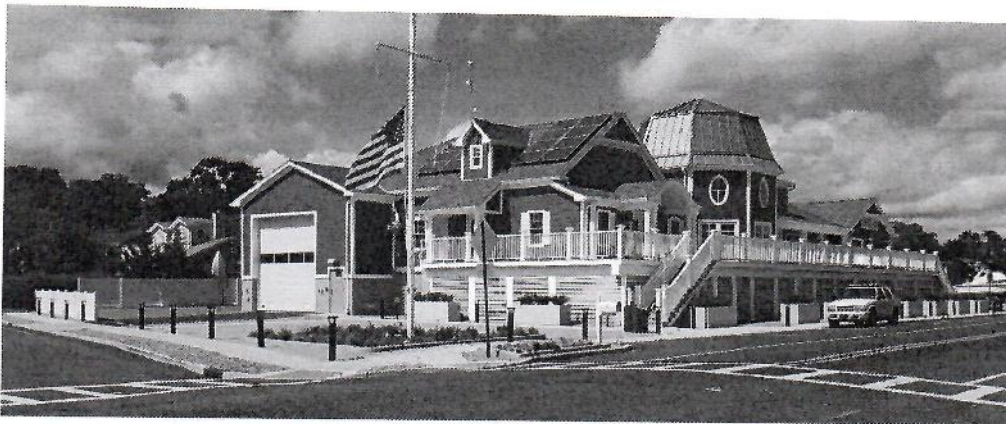
Figure 1: The newly-completed Shark River Municipal Marina building
