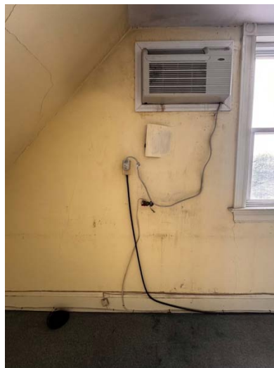
Electrical in this room is limited to junction boxes mounted to baseboards with un-enclosed electrical wires running between them. The room is unheated. (A non-conforming A/C unit was installed by cutting a non-conforming hole in the south wall sometime in the 1980s).
