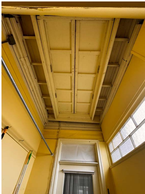
Looking up at the existing 2 nd floor side porch floor. Note the pitch of the support boards running left to right. Also visible are the underlying floorboards of the original porch.
