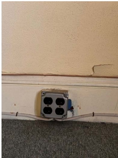
Electrical in this room is limited to junction boxes mounted to baseboards with un-enclosed electrical wires running between them. The room is unheated. (A non-conforming A/C unit was installed by cutting a non-conforming hole in the south wall sometime in the 1980s).
