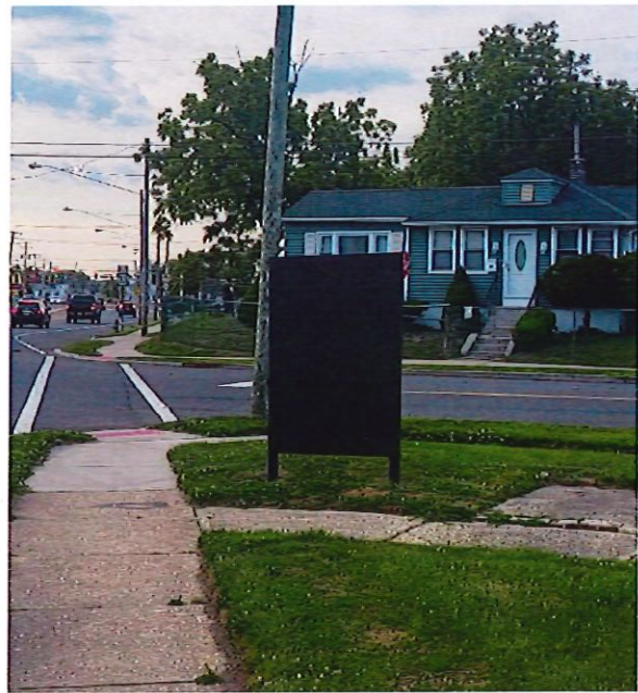
Rec board – Rt 35 and 9 th Ave. (Bradley Park)
