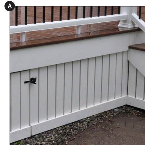
VERTICAL SLAT DECK SKIRT 1"X4" PRESSURE TREATED DECK BOARDS WITH 1/2" SPACING PAINTED SIMPLY WHITE BY BENJAMIN MOORE
