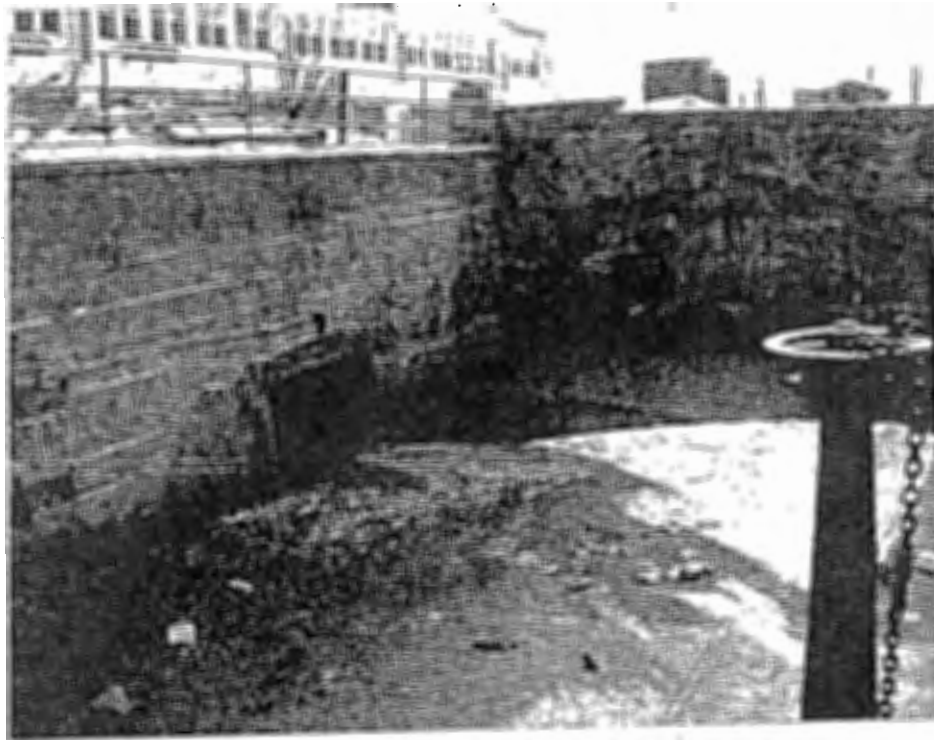
Photo #3 - View of Headwall at East End of Lake.
