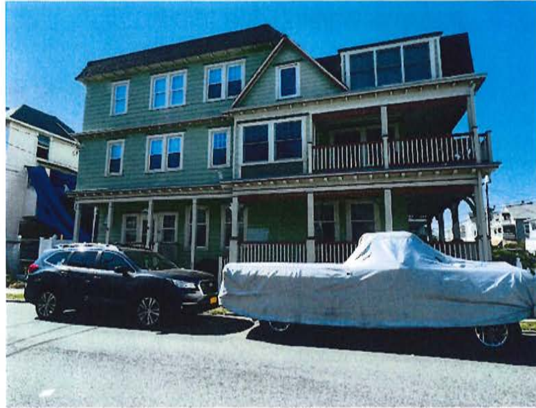
east elevation (note gable from nineteenth-century building, three story addition to south with false mansard on east side only, and third-floor, gambrel addition to north); note some peeling paint and irregular board on second and third floor clap to the rear
