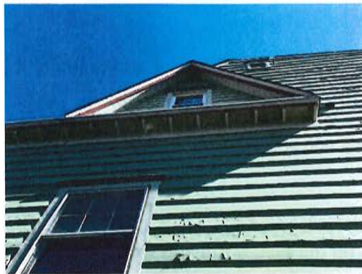
nineteenth-century west gable and juncture of early twentieth-century addition
