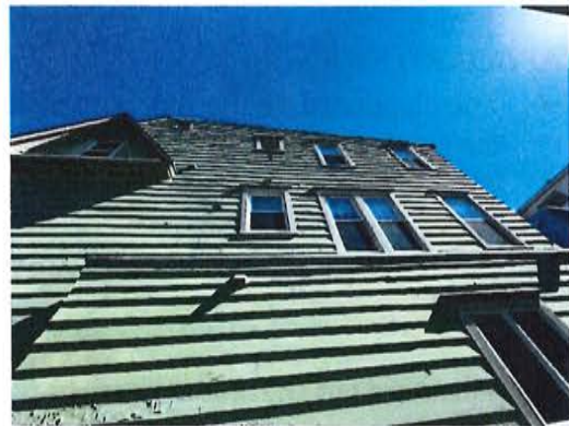
upper rear west wall
